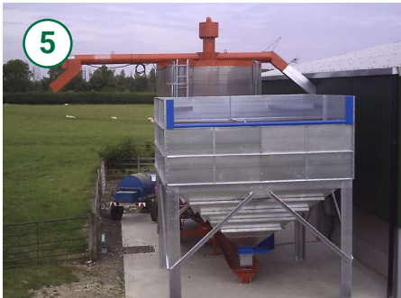
5 A 38 ton dryer fitted with twin horizontal discharge to allow lorries to be filled or grain to be emptied into a storage bin.
