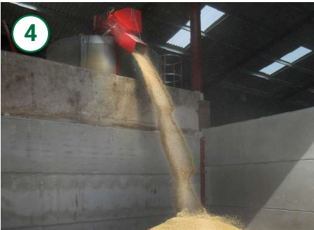
4 Discharging over a grain wall provides unrestricted unloading capacity. Dry grain can then be moved to permanent storage with a telehandler or loaded for sale.
