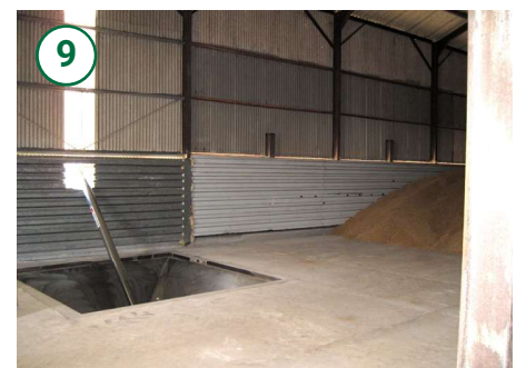
9 Reception pit allows tipping straight from the field or filling with the handler from a wet grain heap.
